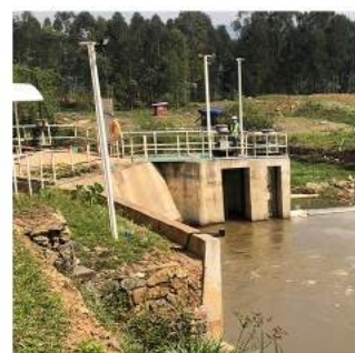
Intake: majority of water is temporarily diverted into the channel
