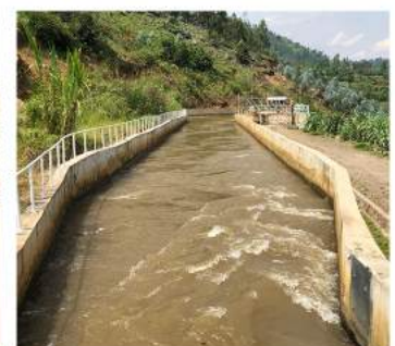
Intake: majority of water is temporarily diverted into the channel
