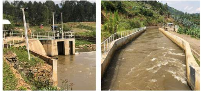
Intake: majority of water is temporarily diverted into the channel
